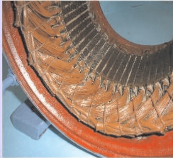
Figure 10: Coils in the stator
