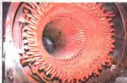
Windings of induction electric motor
