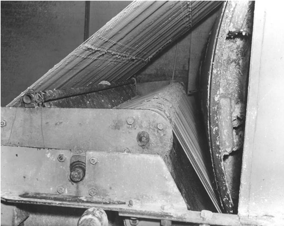
Figure 7.20. String discharge mechanism on a filter handling silica gel
