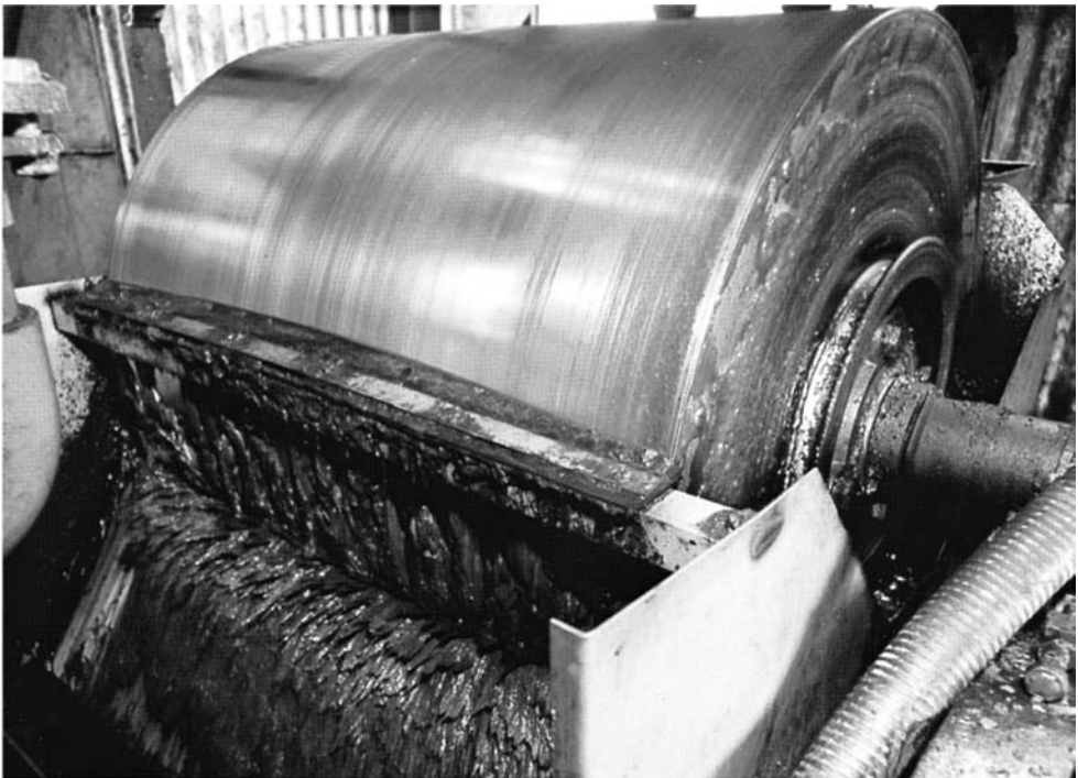
Figure 1.44. A wet drum separator in action
