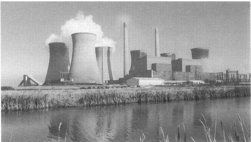
Figure 13.14. Natural draught water-cooling towers
