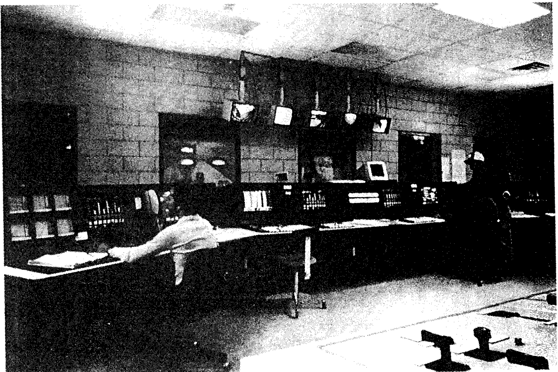
FIGURE B.9 Typical control room with computer control. (Courtesy of Honeywell .)
