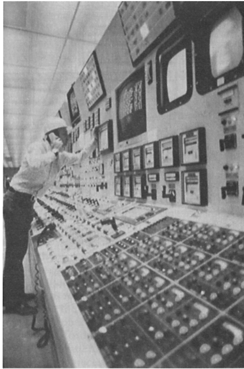
FIGURE 1 Long panelboard containing indicators and controllers used in large processing plant. Generally this type of panel was used in the early 1970s. The very beginnings of the cathode-ray tube (CRT) displays for annunciators are indicated by the CRTs in the upper right-hand portion of the view.
