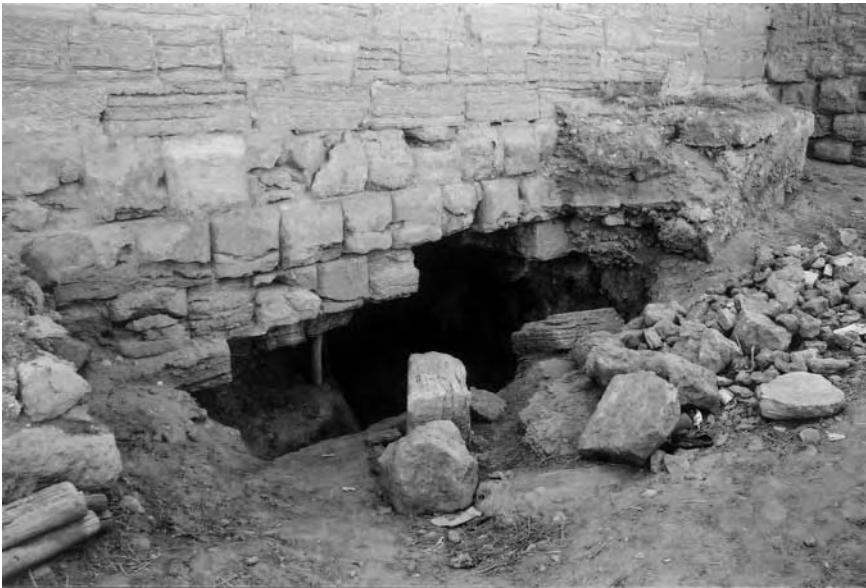
Figure 4.29 One of the mines built by the Sasanians under the west wall at Dura Europos and the assault ramp adjacent to tower 15.
