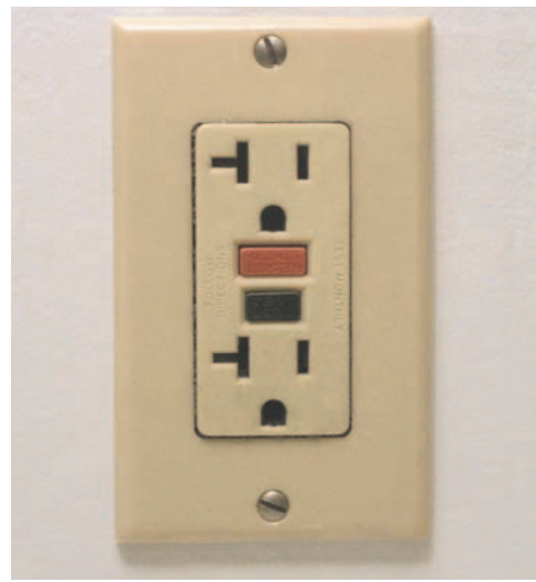
Figure 3–3 Ground fault interrupter.
