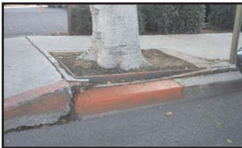
This sycamore tree has outgrown its planter and is damaging the sidewalk and curb.
