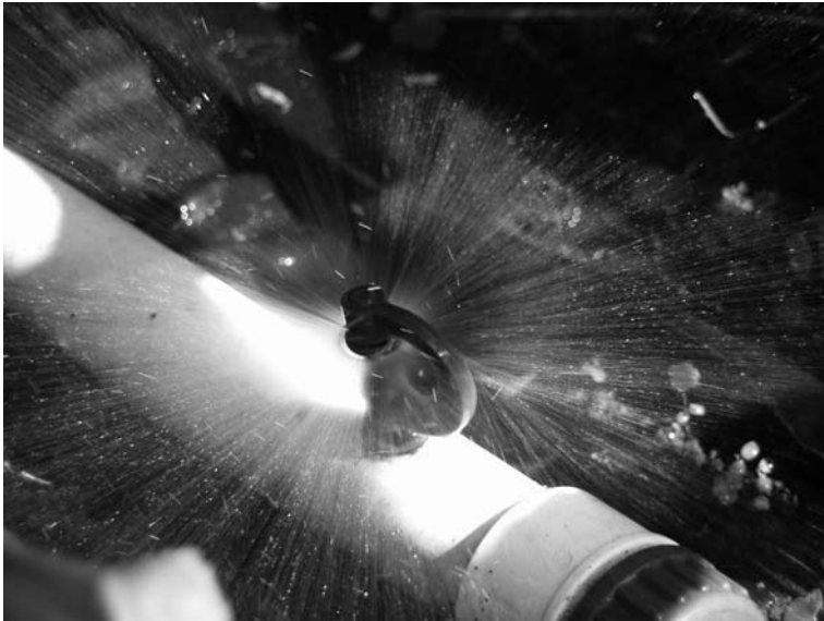
Picture 15.2 Low level sprinkler irrigation used with strip irrigation of soil grown crops
