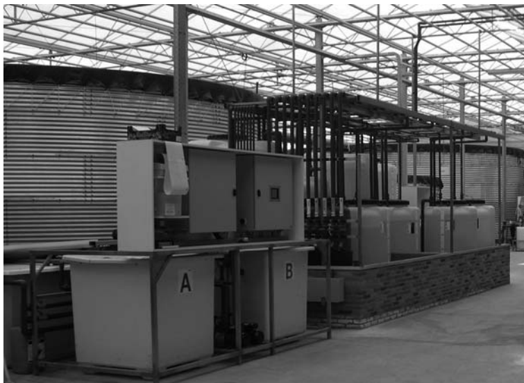
Picture 12.1 Installation for the preparation of nutrient solutions. At the back the reservoirs for concentrated fertilizer solutions are placed
