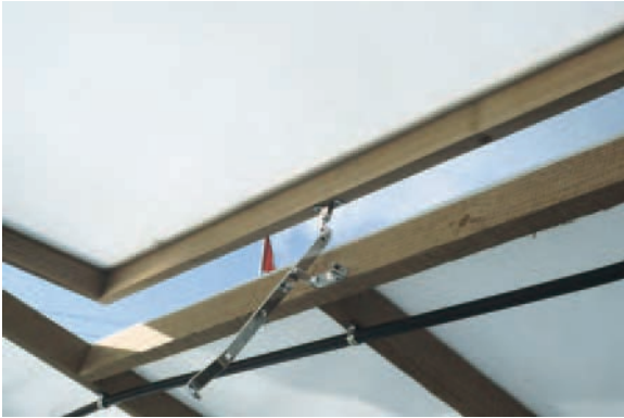
Figure 25: A simple greenhouse roof vent.
