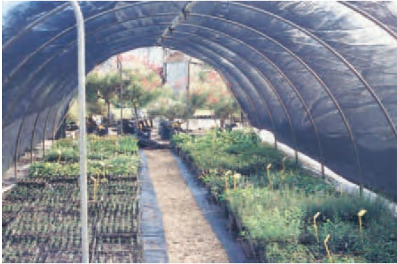
Figure 29: A simple tunnel shadehouse. These are available in kits and are easy to construct.
