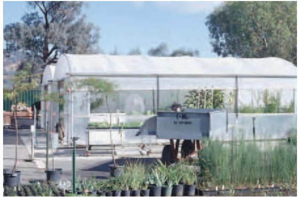
Figure 26: Plastic-clad greenhouses are widely used in horticulture as they are the least expensive greenhouse structure to build.
