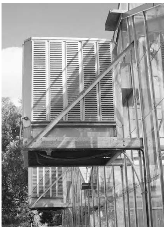
Figure 11.4: Evaporative coolers are used to cool greenhouses and glasshouses.
