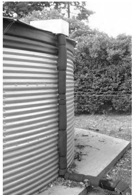
Figure 10.1: In areas with sufficient rainfall, rainwater can be stored in tanks. This method of supplying water may involve higher initial costs but in the long term can be cheaper than buying water.
