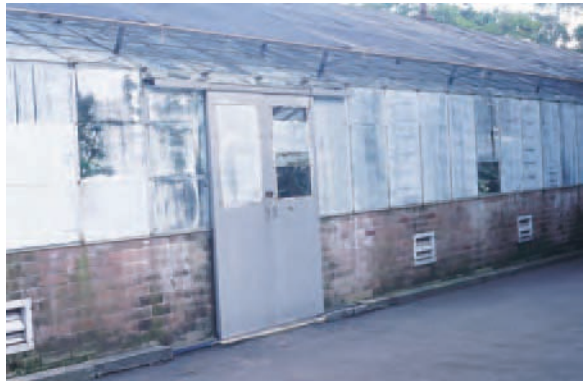
Figure 30: The panels of this glasshouse have been whitewashed to reduce light transmission during a hot spell. The whitewash can be removed easily when the weather cools.
