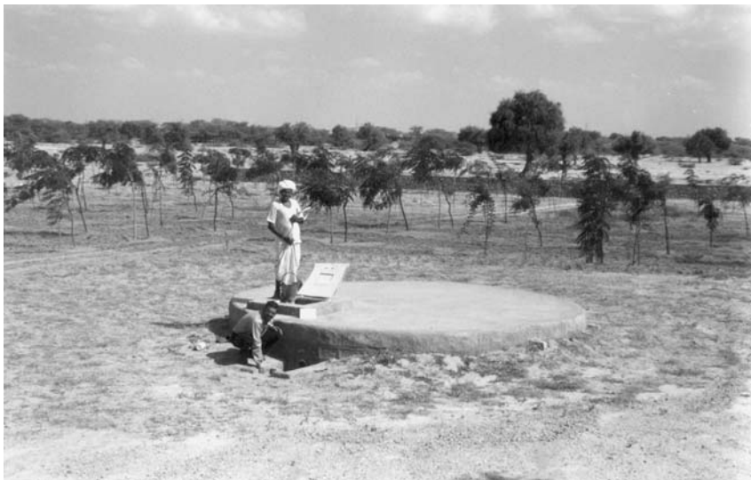
Figure 23.5 A Tanka—a common household rainwater harvesting system in Rajasthan, India.
