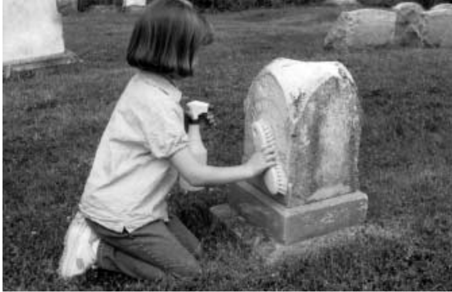
Often after simply training and with proper supervision, even young volunteers can be used to clean headstones. Here a young volunteer uses water and a natural bristle brush to do the initial cleaning.
