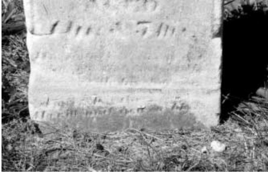
An infill repair is done not only to improve appearance but to reinforce a repair. Here the repair is done so that the finished edges are of the same worn appearance as the rest of the marker. From a few feet away the repair is indiscernible.
