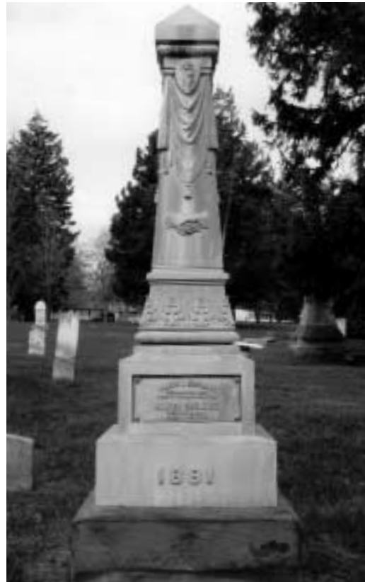
Zinc monuments, because of their unique characteristics, have deteriorated very little over time.
