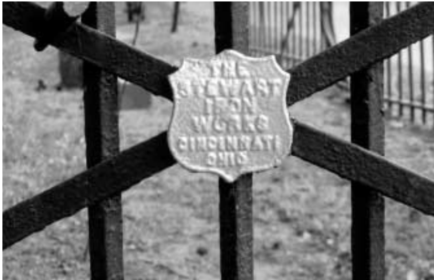
In some instances the original company nameplate will remain on the wrought iron fence. This information is valuable when trying to replace or repair fence sections.
