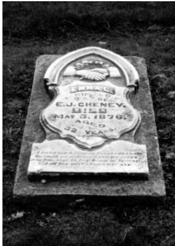
Setting broken markers in cement is not an acceptable practice, but removing stones that have been set in concrete is too risky.
