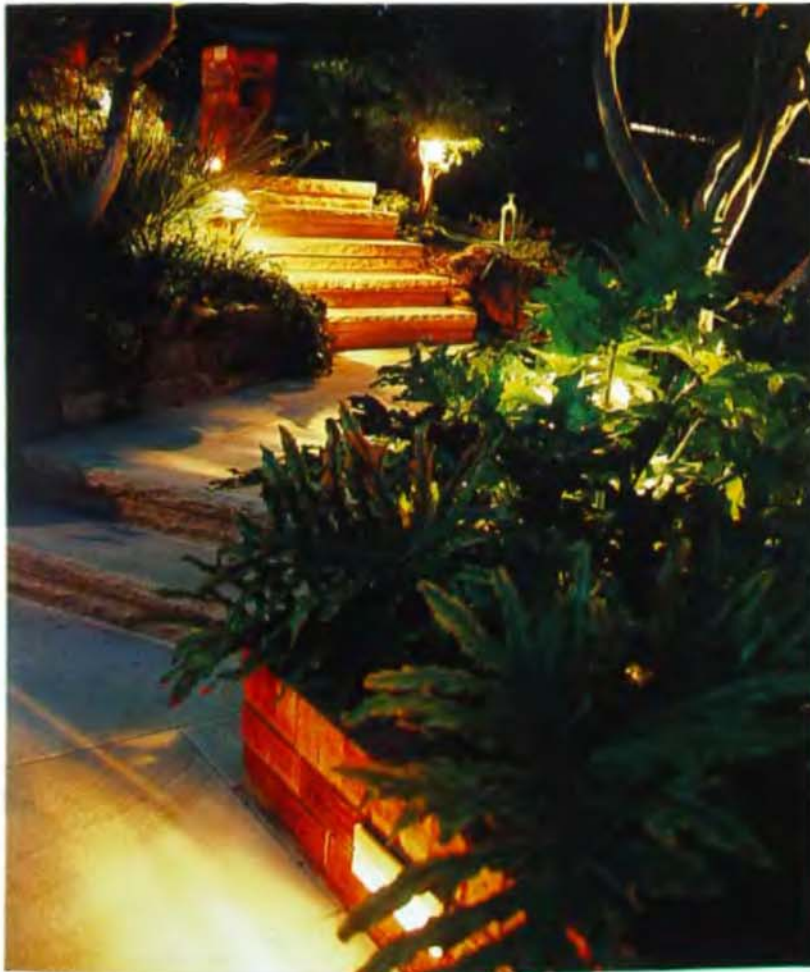
left: Recessed bricklights illuminate the path while stem-mounted luminaires light the steps upwards. Some uplighting of small trees adds interest.
