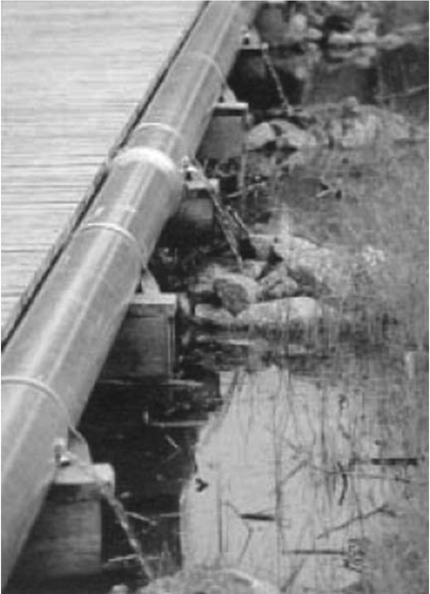
Figure 6.10. A surface flow wetland system in the U.S. (courtesy of USEPA).
