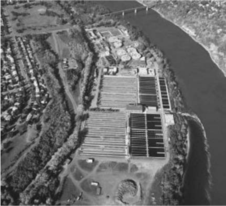
Figure 7.2. An aerial photo of Goldbar Wastewater Treatment Plant in Edmonton, Alberta, Canada.
