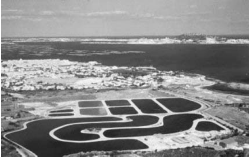
Figure 6.1. A waste stabilization pond system in Mèza, France. It contains two small anaerobic ponds, four experimental facultative ponds, and one series pond system composed of a facultative pond and four maturation ponds.
