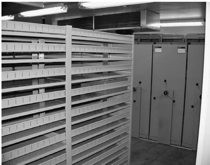
Fig. 17.10. The inside of OPGC medium-term storage cooler maintained at 2°C–5°C and 30% relative humidity.
