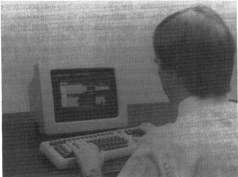
Figure 4-12. Keyboard Used to Access EMS (Photo Courtesy Control Systems International)
