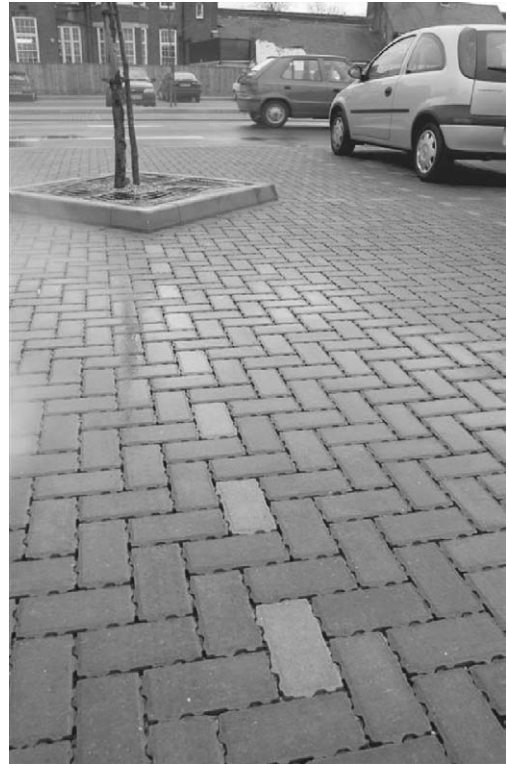
FIGURE 10.4 Permeable segmental paving.
