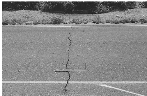
FIGURE 8.8 Thermal cracking.
