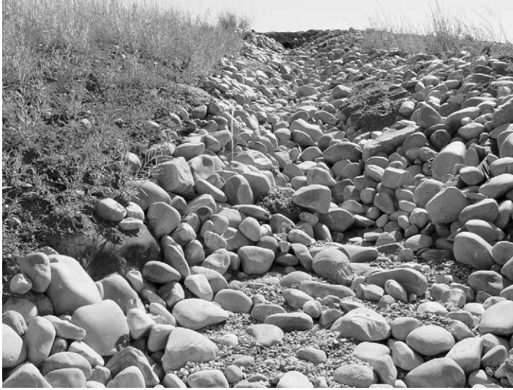
FIGURE 13.3 Rock-lined ditch.
