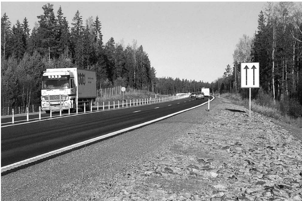
FIGURE 4.1 A Swedish “2 + 1” rural arterial, divided by flexible barrier (Source: Larsson et al., 2003).
