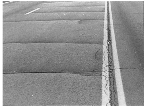
FIGURE 8.13 Reflection cracking.
