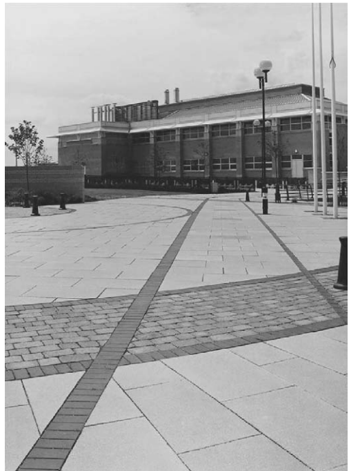
FIGURE 10.2 Precast concrete pavers and paving flags.
