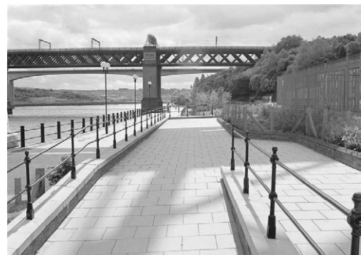
FIGURE 10.5 Footpath surfaced with concrete paving flags.
