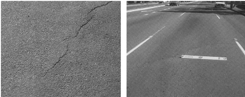
FIGURE 19.14 Diagonal cracks in flexible pavements (Source: Austroads, 1987).
