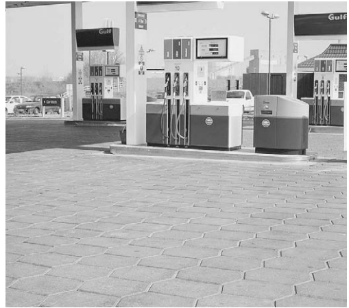
FIGURE 10.3 Segmental paving used to resist petroleum spillages.
