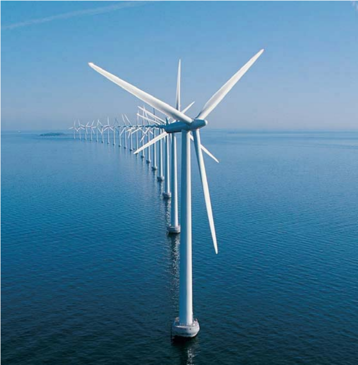
Fig. 4.26. Middelgrunden offshore wind farm, Denmark (Courtesy of Siemens Wind Power A/S, www.siemens.com/powergeneration )
