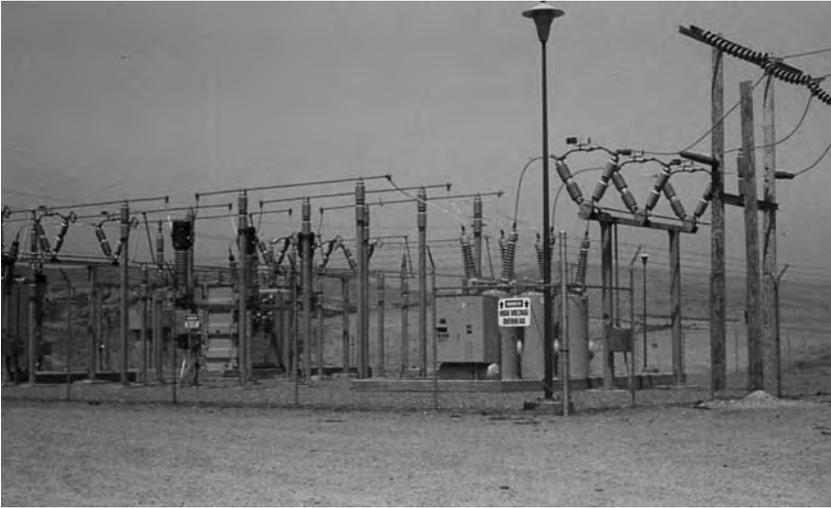
**Figure 6.10** Distribution substation. (Courtesy of Marshal F. Merriam.)
