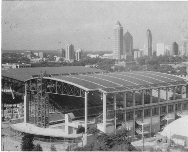
FIGURE 3-8 Roof (pv) of Atlanta's Aquatic Center with 345 kW grid-connected power system. (Source: Georgia Institute of Technology. With permission.)
