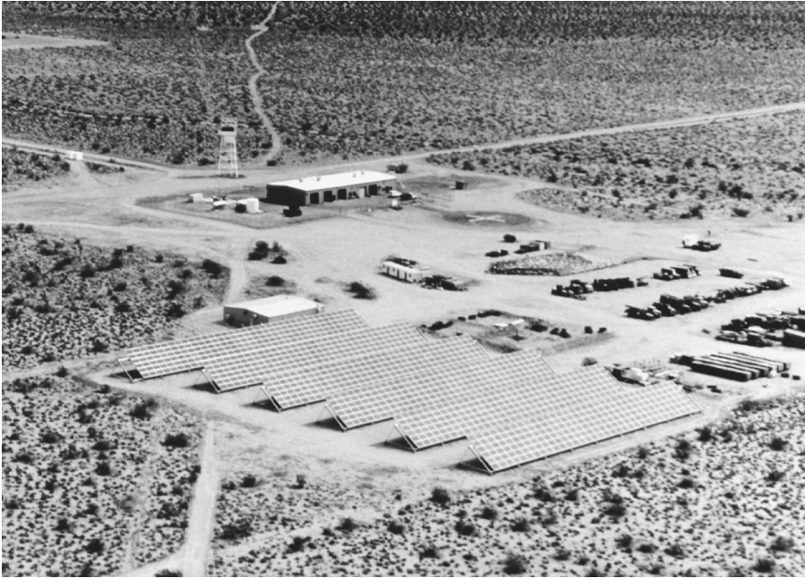
FIGURE 12-6 A 300 kW photovoltaic-diesel hybrid system in Superior Valley, California. (Source: ASE Americas Inc., Billerica, MA. With permission.)
