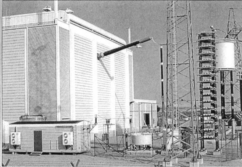
Fig. 6.79 Active DC filter at the Swedish terminal of the Baltic cable link. (Courtesy of ABB, Sweden.)
