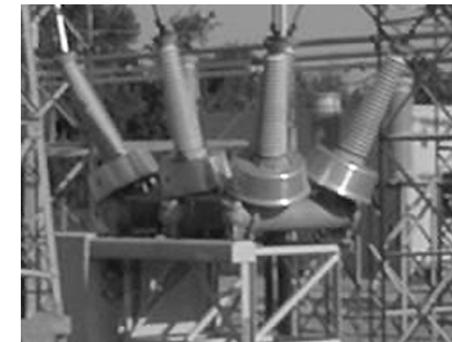
FIGURE 2.6.28 High-voltage circuit breaker with BCTs mounted underneath a metallic cover. (Photo courtesy of Kuhlman Electric Corp.)
