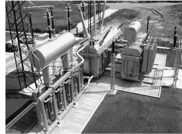
FIGURE 2.3.14 Quadrature booster set (300 MVA, 50 Hz, 400 \pm 12 \times 1.25\% / 115 \pm 12 \times 1.45\% kV).
