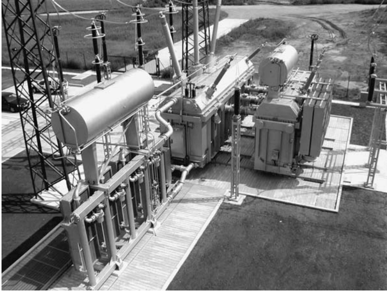
FIGURE 2.3.14 Quadrature booster set (300 MVA, 50 Hz, 400 \pm 12 \times 1.25\% / 115 \pm 12 \times 1.45^\circ kV).
