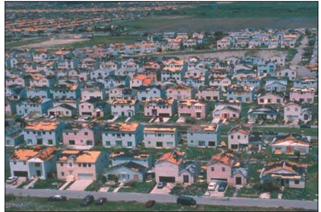
Hurricane Andrew, one of the most destructive hurricanes in US history, inflicted widespread damage
